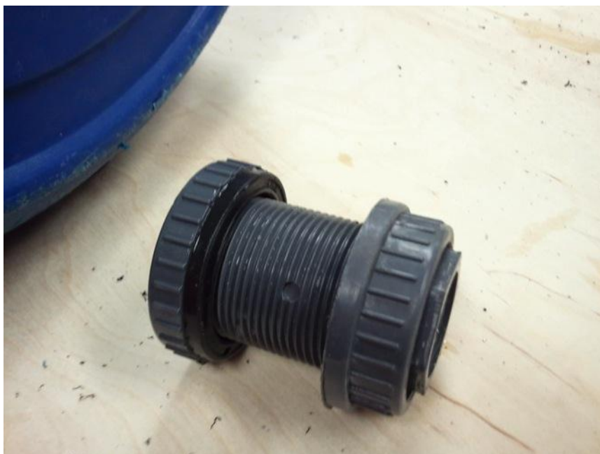
Insert and secure the bulk head fitting
